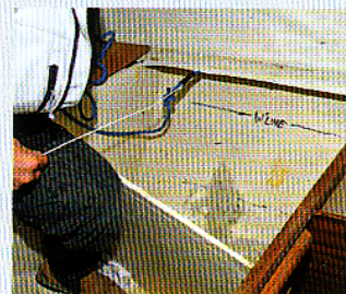
We poked out our hauling line using a straightened coat hanger
